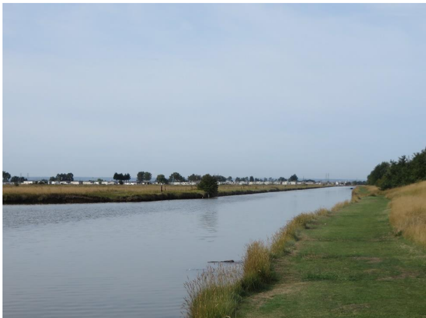
Queenborough Lines, Sheerness
