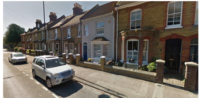
Typical house type on Stone Street, presenting opportunity for the greening of private gardens
